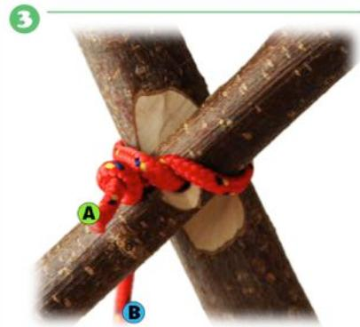
Execute a simple knot and move it near the joint. Then, tighten by pulling the opposed end of the cord (B).
